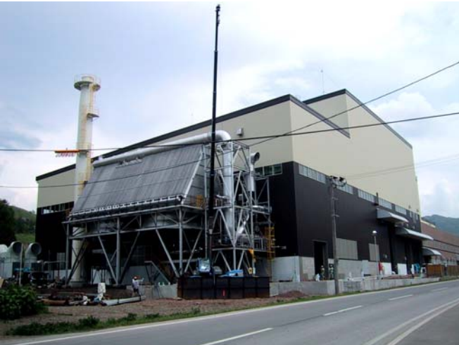
Complete view of the structure (Stack side)
