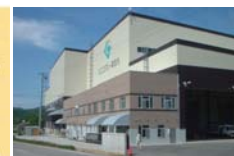
Hitachi Metals 200 tpd PDMR Facility in Utashina, Japan
